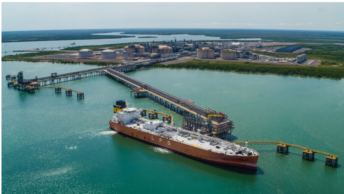
The Project's first LPG shipment undertaken by the LPG carrier "Hellas Gladiator"
