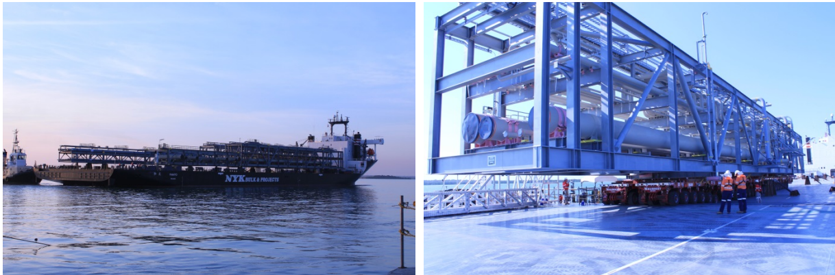
Module unloading at MOF at Bladin Point, Darwin
