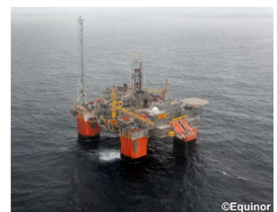
©Equinor Snorre Project's offshore production facility (Norway)
