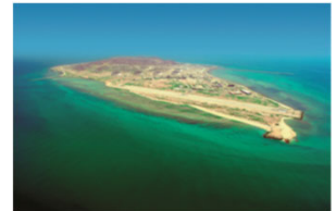
Abu Dhabi Offshore Oil Fields Zirku Island (oil processing facility)
