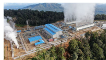
Rantau Dedap Geothermal Power Plant (Indonesia)
