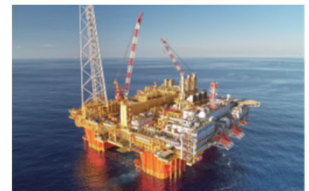
Ichthys LNG Project CPF (Central Processing Facility)
