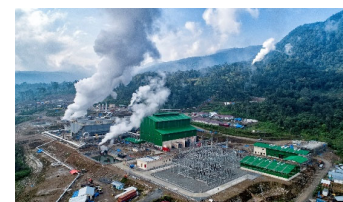
Muara Laboh Geothermal Power Plant (Indonesia)
