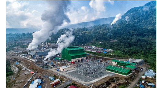
Muara Laboh Geothermal Power Plant (Indonesia)
