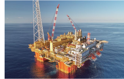
Ichthys LNG Project CPF (Central Processing Facility)
