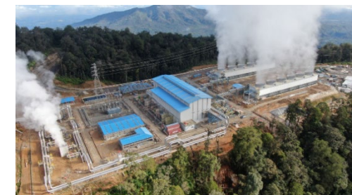
Rantau Dedap Geothermal Power Plant (Indonesia)
