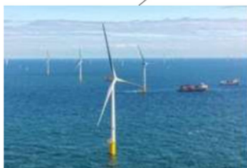
Borssele III/IV offshore wind farm
