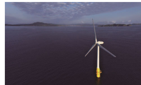
Image of floating offshore wind power project (Photo by Mr Hoichi Nishiyama)
