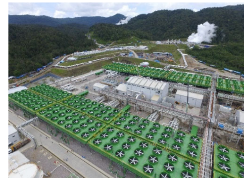
Sarulla Geothermal Independent Power Producer (IPP) Project
