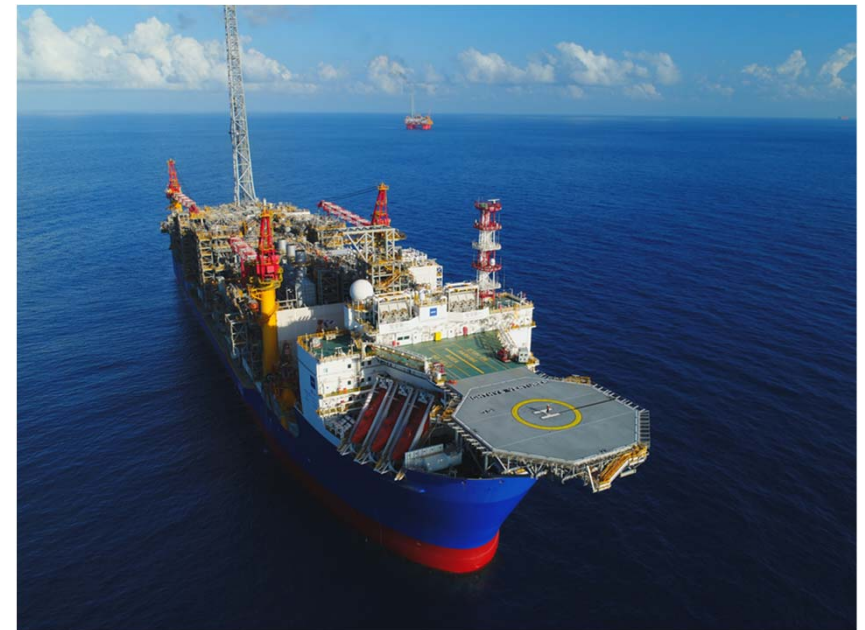
FPSO at Ichthys Gas- condensate Field
