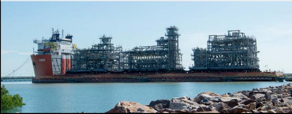
Completion of off-loading of the final onshore module (Aug/2016)
