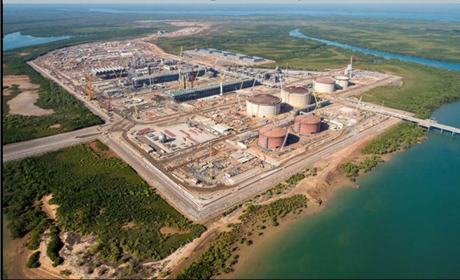
Construction of LNG plant (Aug./2015, Darwin)
