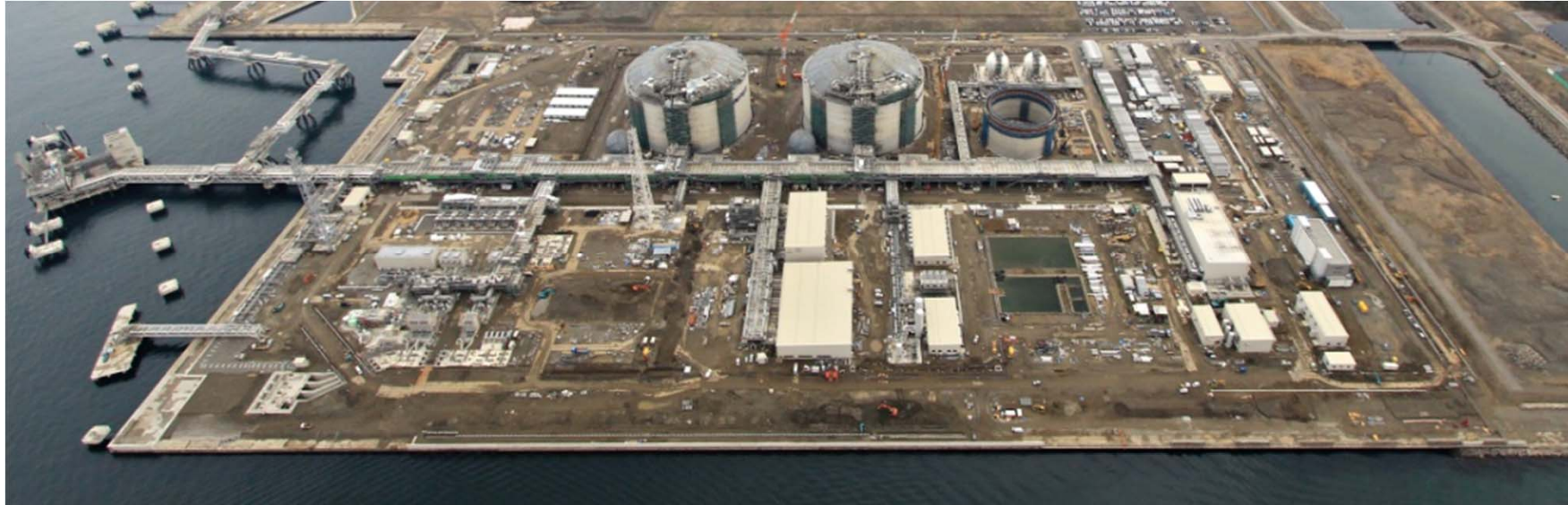
(Full view of Naoetsu LNG Receiving Terminal, as of April 2013)
