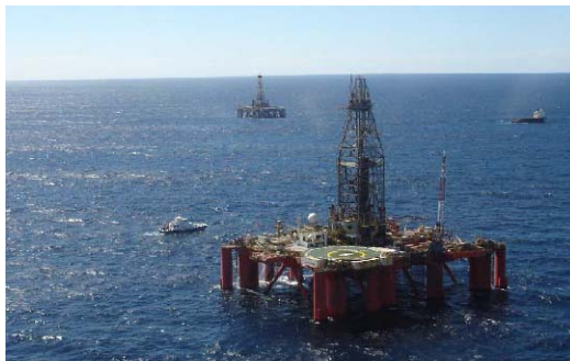
Drilling Rig (Van Gogh Oil Field)
