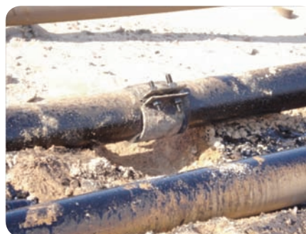
Treating an oil leak in Egypt
