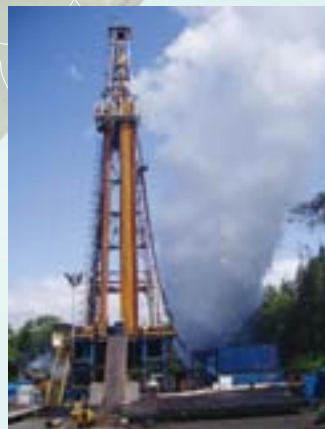
Fumarolic testing at a geothermal well (Teiseki Drilling Co., Ltd.)
