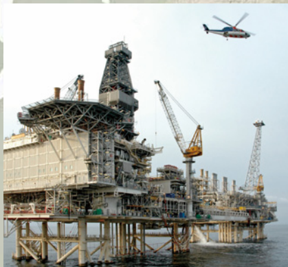
Marine production facilities
