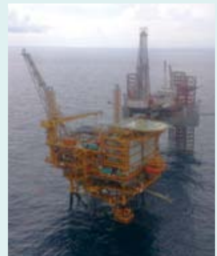
Offshore production facility in the Ruby Gas Field
