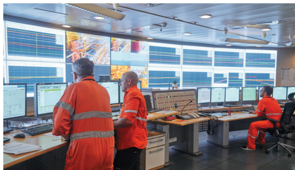
Control center inside the CPF
