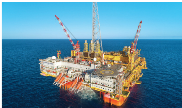
Offshore production and central processing facility (CPF)
