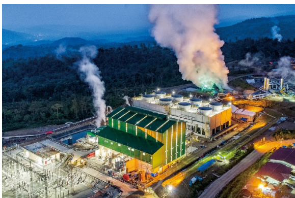
Muara Laboh Geothermal Power Plant
