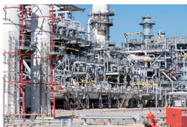
Onshore gas liquefaction plant
