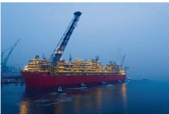
The Prelude FLNG facility
