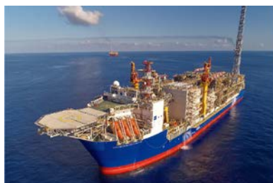
Floating Production Storage and Offloading (FPSO) facility (“Ichthys Venturer”)
