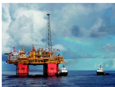
Central Processing Facility (CPF)
