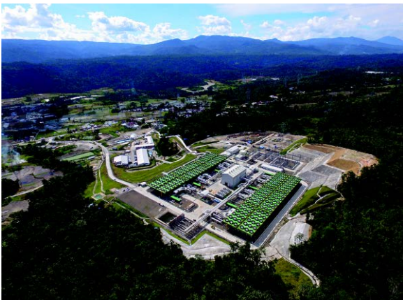
First power plant of Sarulla geothermal power generation project
