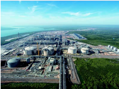
Onshore gas liquefaction plant (Darwin)
