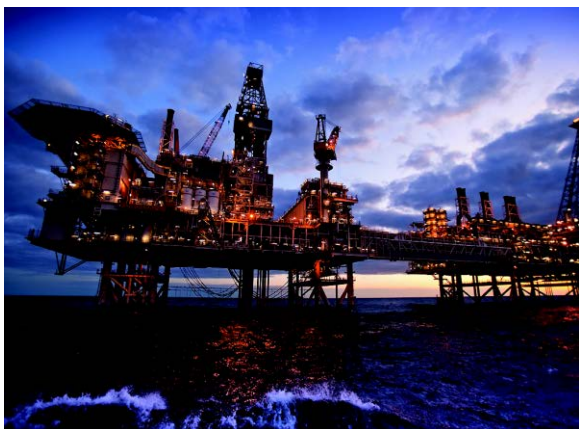
ACG Oil Fields offshore production facilities
