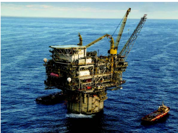
Offshore production facilities of the Lucius Field
