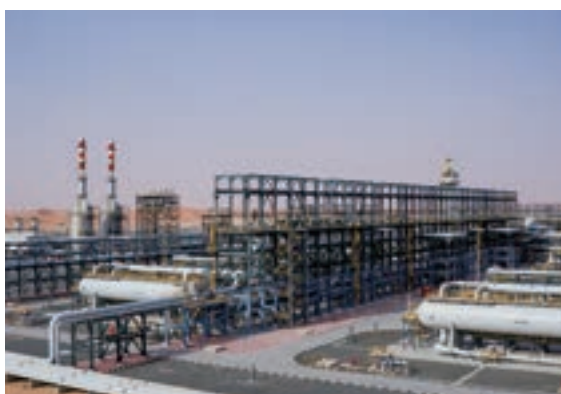
Oil processing facility
