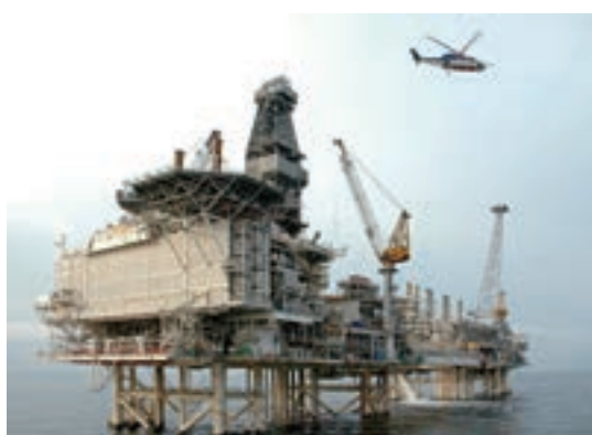
Offshore production facility
