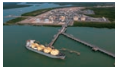
Ichthys onshore production plant
