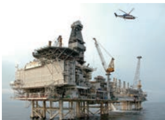
Offshore production facility
