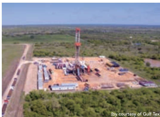
Drilling operations site
