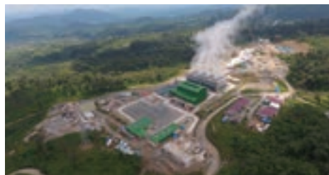
Muara Laboh Geothermal project
