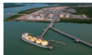
Ichthys onshore production plant
