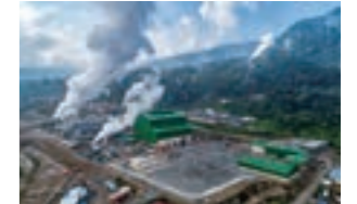
Muara Laboh Geothermal Power Project
