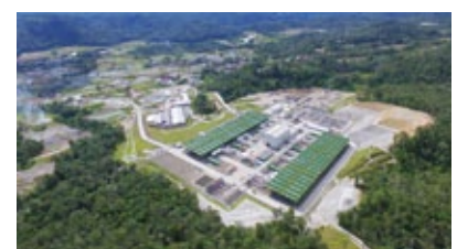
Sarulla Geothermal IPP Project
