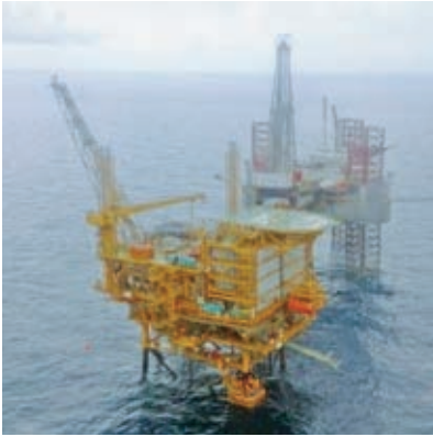
Offshore production facility in the Ruby Gas Field
