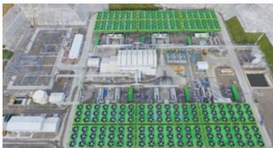
Commercial operations commenced at the first unit of the Sarulla Geothermal Independent Power Producer (IPP) Project
