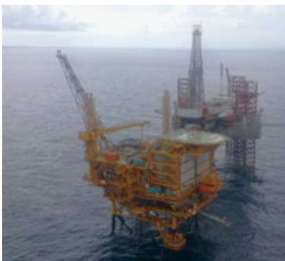
Offshore production facility in the Ruby Gas Field
