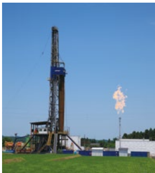
Drilling work at the Minami-Nagaoka Gas Field (Nagaoka City, Niigata Prefecture)
