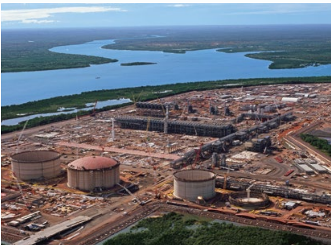
Steady progress in construction of the onshore LNG plant
