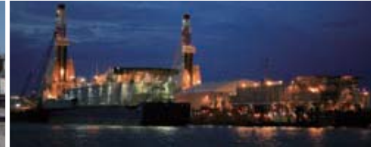
Kashagan Oil Field (offshore facility)
