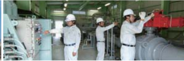
Inspecting for leaks at a valve station
