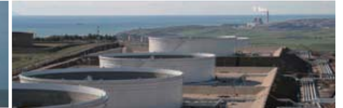
BTC Pipeline (Ceyhan Terminal)
