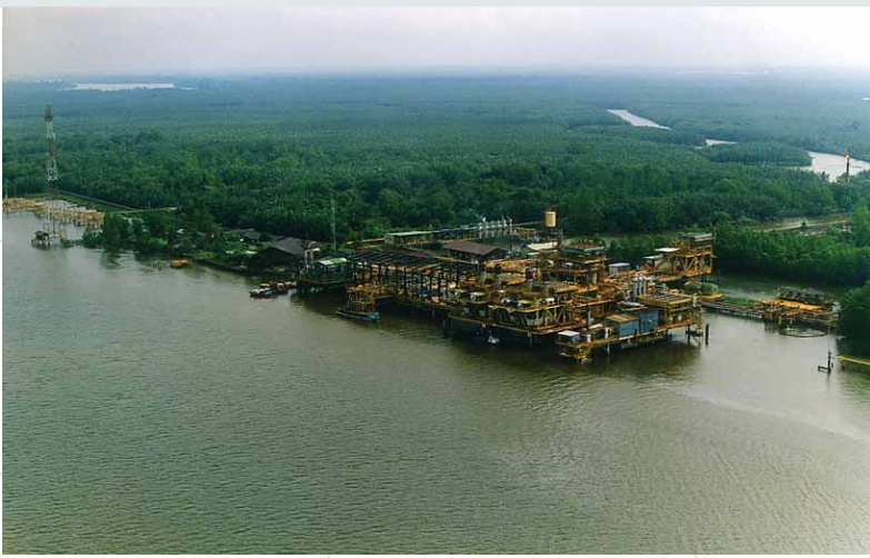
Handil Central Processing Area
