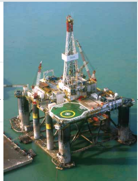
Drilling Rig, WA-285-P
