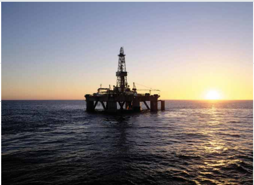
Drilling Rig, Timor Sea
