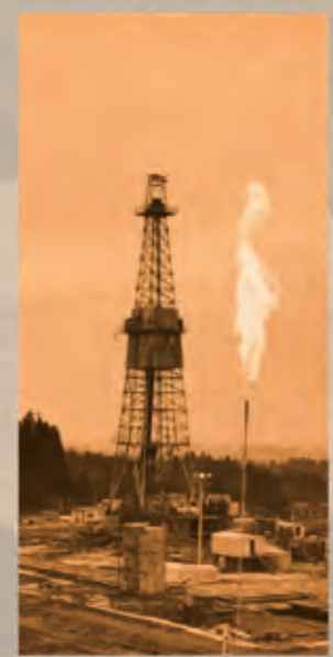
Photo: Shin-Sekihara Well No.4 undergoing a natural gas production test in 1979
